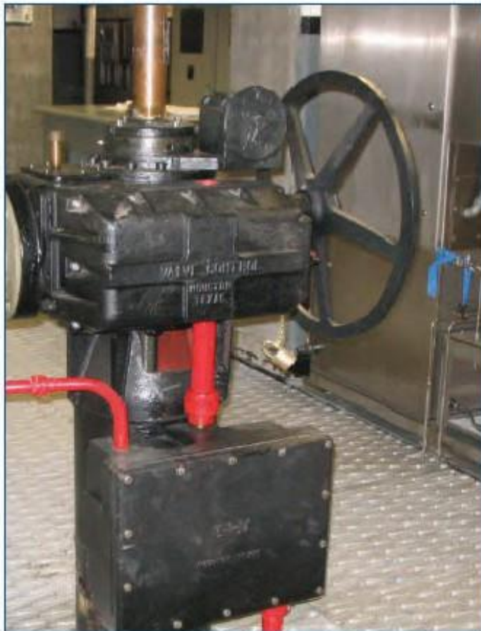
Current M2CP units evolved from proven technology—as shown by this actuator, still operating after more than 50 years at a water distribution and storage system in New York City.
